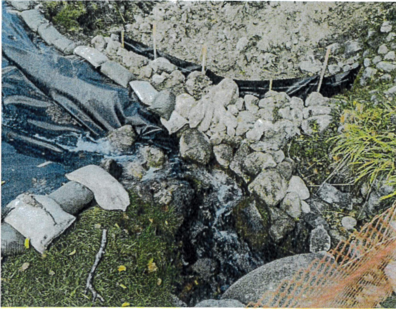
Photo 3. Downstream culvert inlet.
