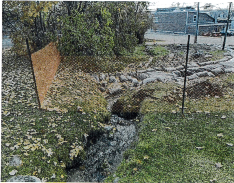
Photo 2. Beginning of stream reroute.
