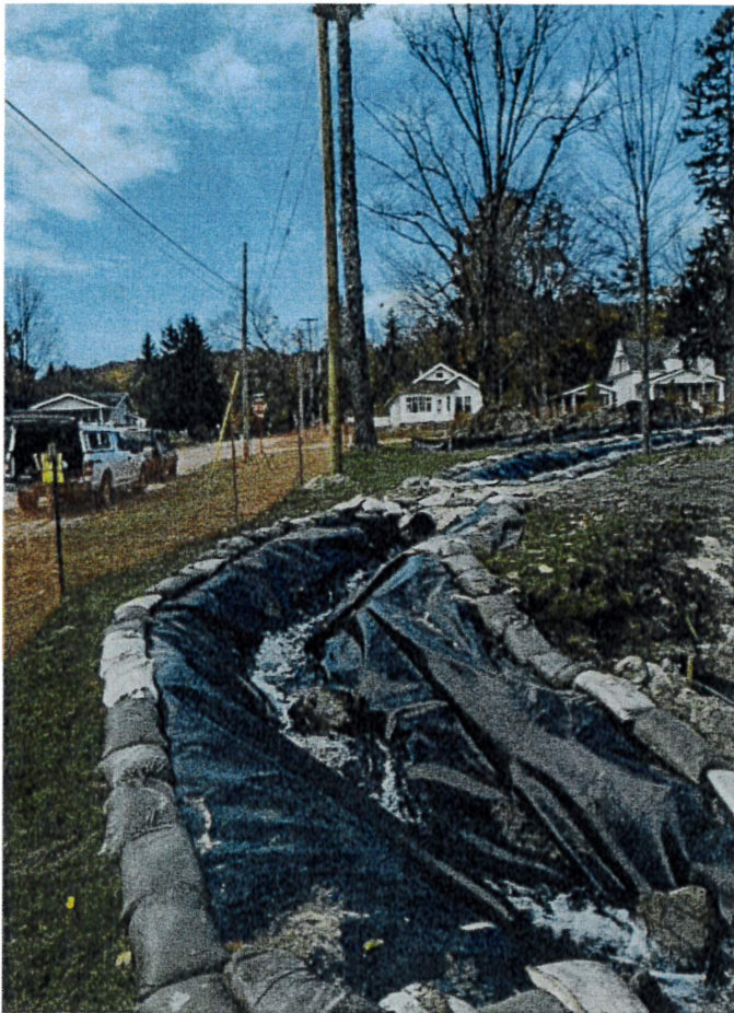
Figure 1. Stream reroute. Photo taken on 10/31/2022.
