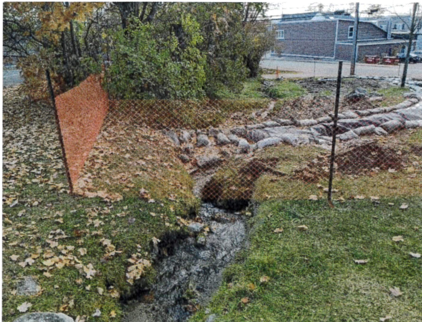
Photo 2. Beginning of stream reroute.
