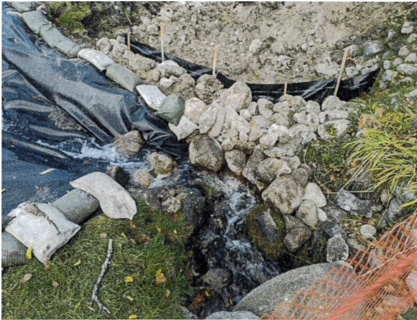
Photo 3. Downstream culvert inlet.
