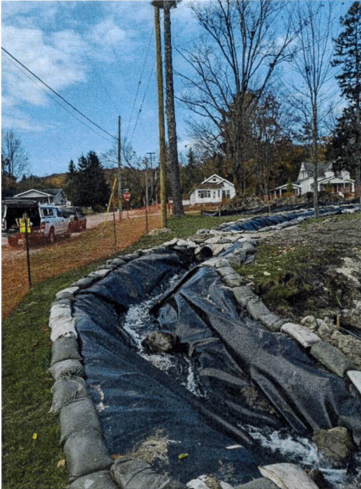
Figure 1. Stream reroute. Photo taken on 10/31/2022.
