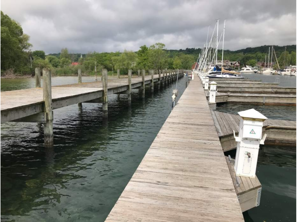
Figure 15: Fixed pier at left; D-Dock (east extent) at right
