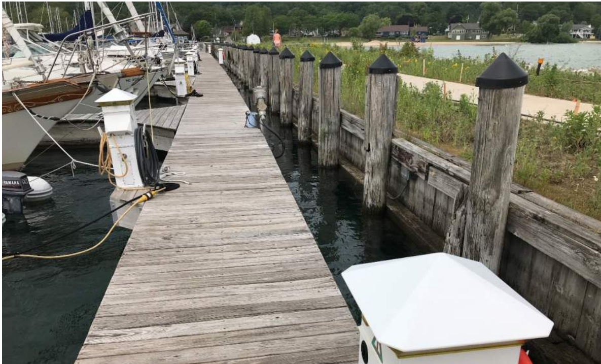
Figure 13: C-Dock with adjacent timber sheeting wall and pathway
