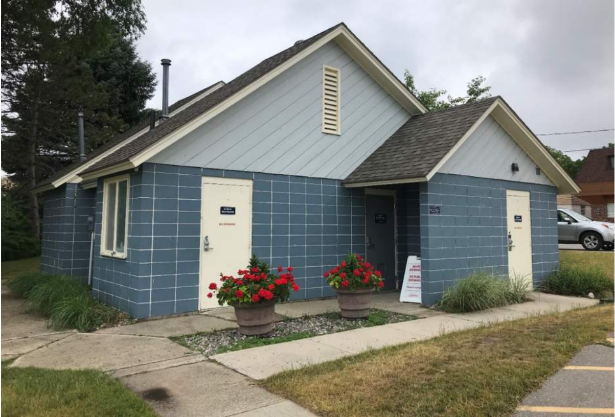
Figure 5: Public restrooms/boater bath house building
