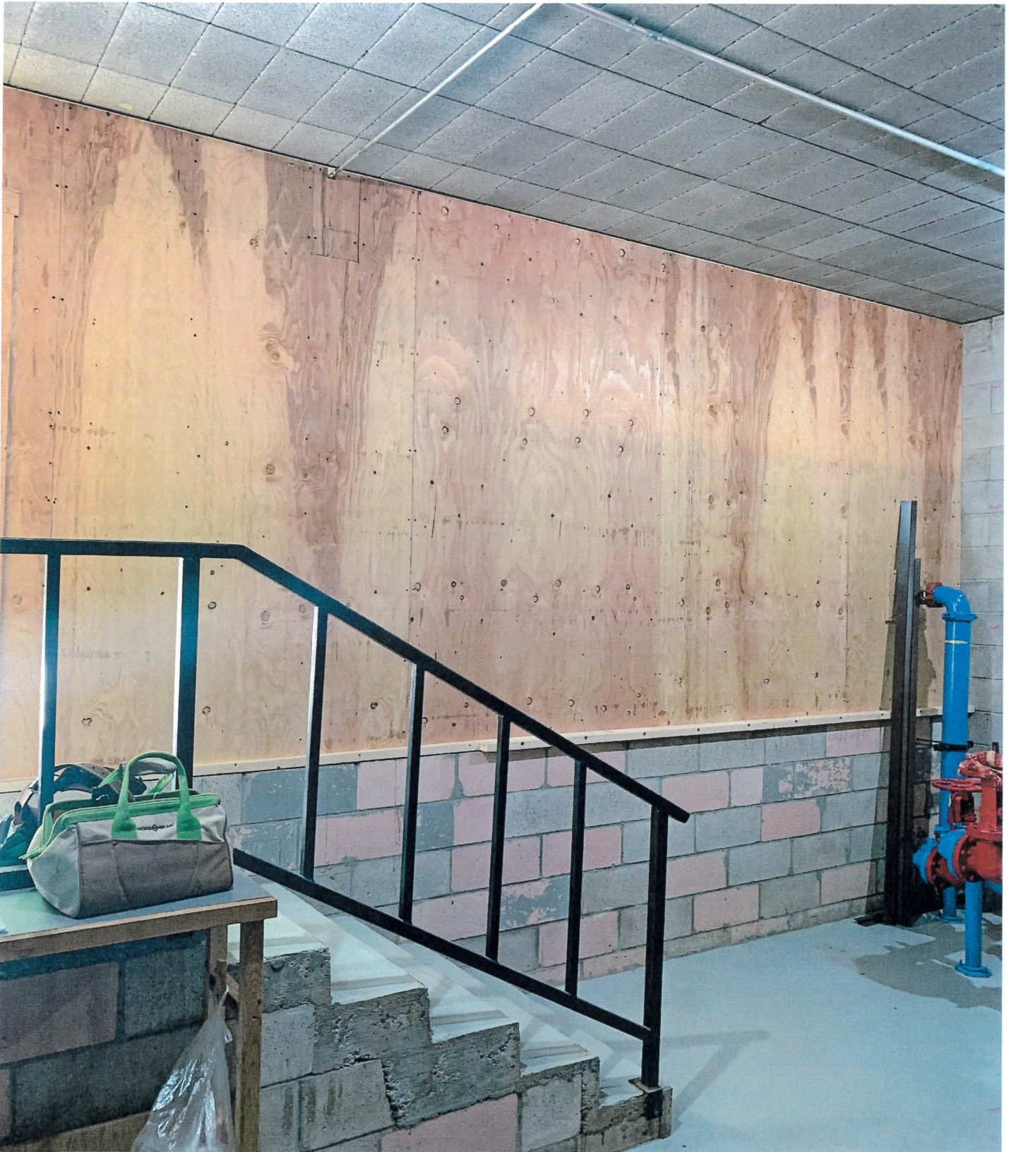
Interior wall insulated and completed, ready for primer sealing.
