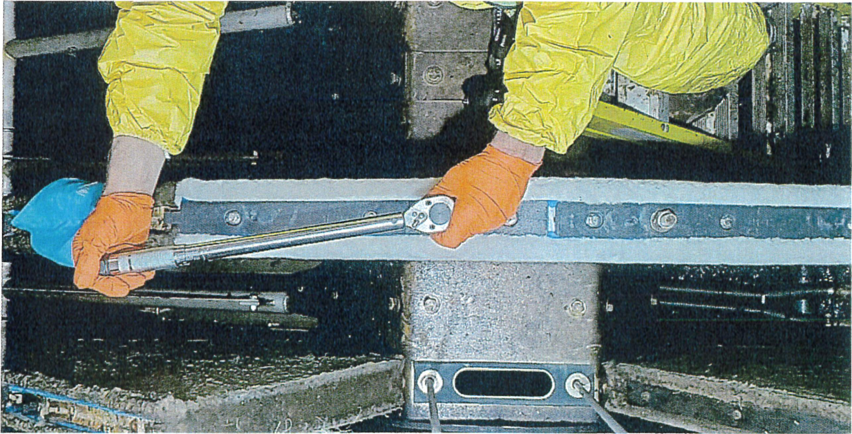
New cloth assembly install, torqued to proper specifications
