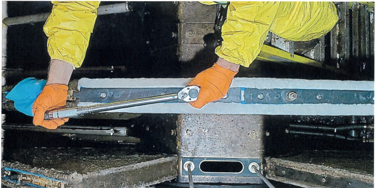
New cloth assembly install, torqued to proper specifications
