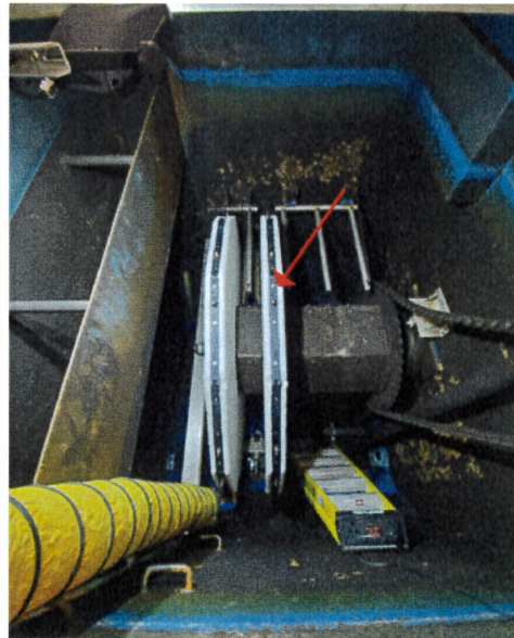
Installed new cloth media
