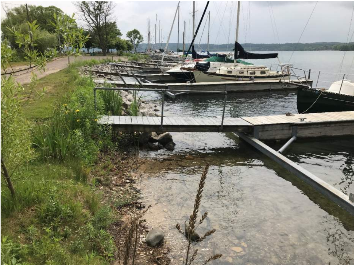
Figure 17: South docks; note stabilized shoreline in background, none in foreground
