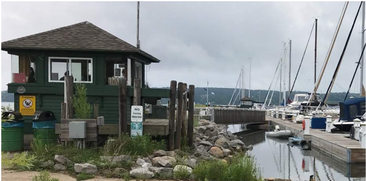
Figure 8: West 'hut' in foreground; B-Dock at right; East 'hut' in background
