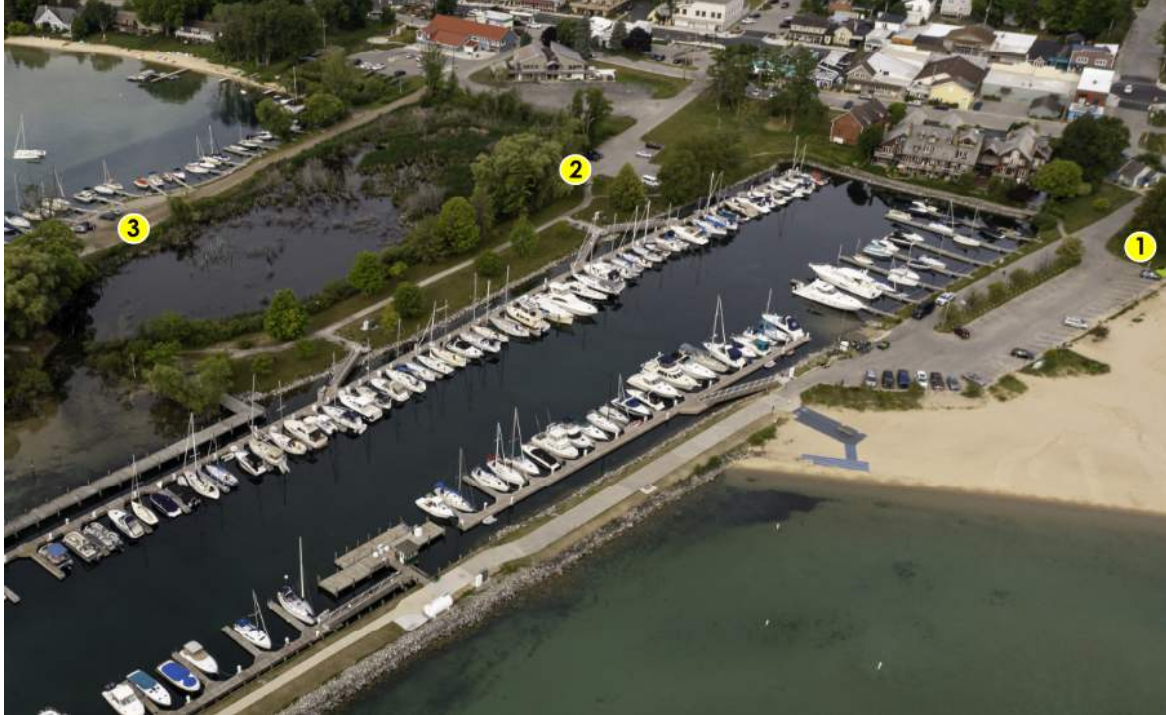
Figure 20: Portable restroom locations (Image credit: Village of Suttons Bay)
