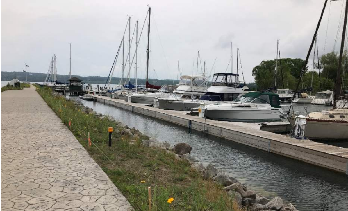
Figure 9: B-Dock, rip rap shoreline, public pathway, native plantings buffer strip to filter runoff
