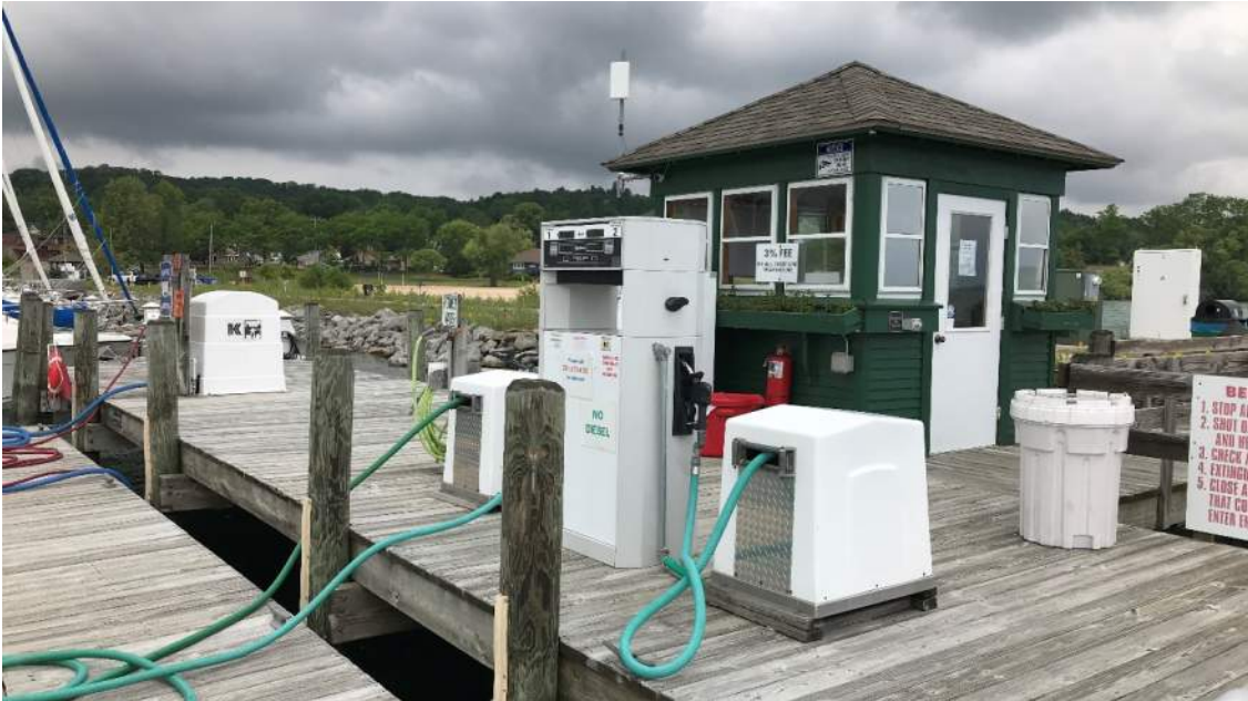
Figure 12: Service pier, fuel dispensers, sanitary pumpout
