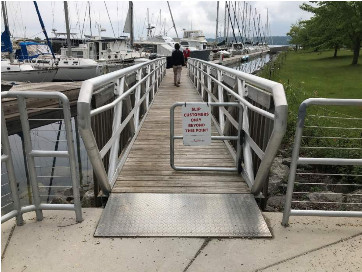
Figure 14: D-Dock gangway and pier in background
