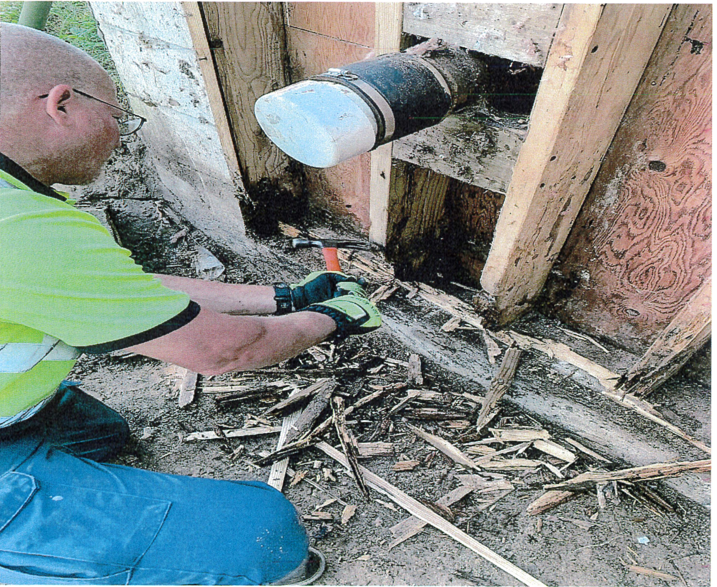
Wall is a total loss, severe damage from runoff infiltrating interior wall.
