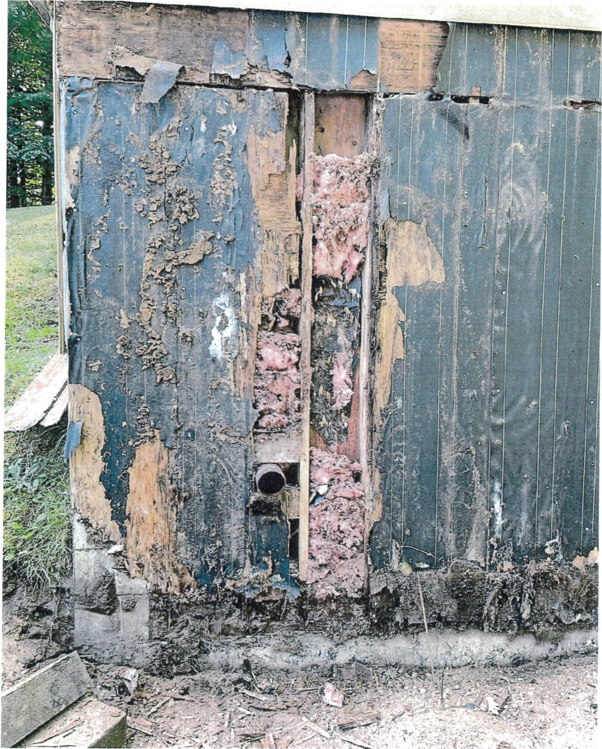
Water damage to exterior wall, mice nests in insulation. Wood completely rotted.
