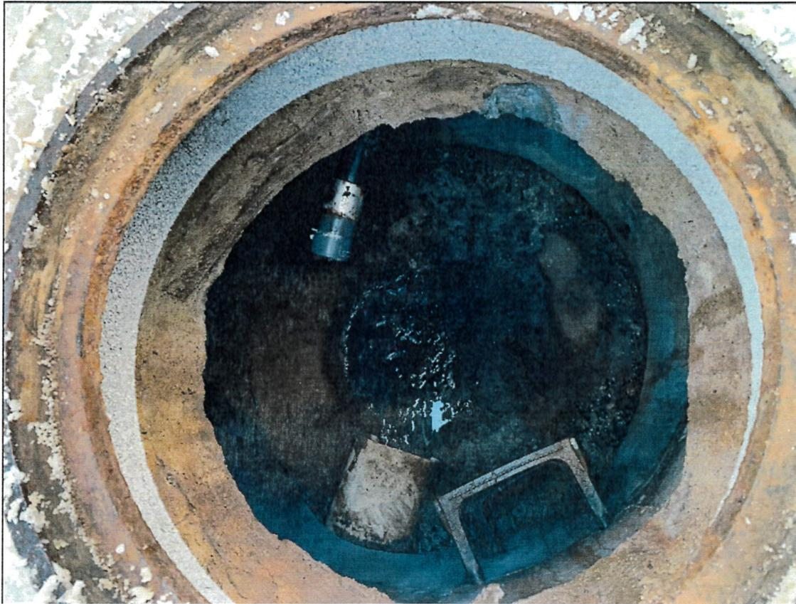
Manhole (MHSN 47) S. Shore Drive before grout and epoxy coating, also inline pipe modification.
