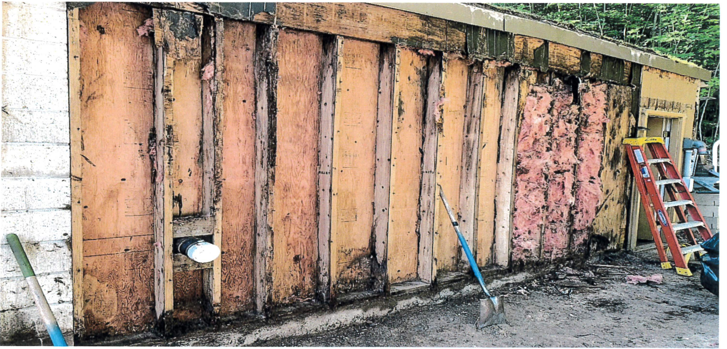
Wall is a total loss, severe damage from runoff infiltrating interior wall.
