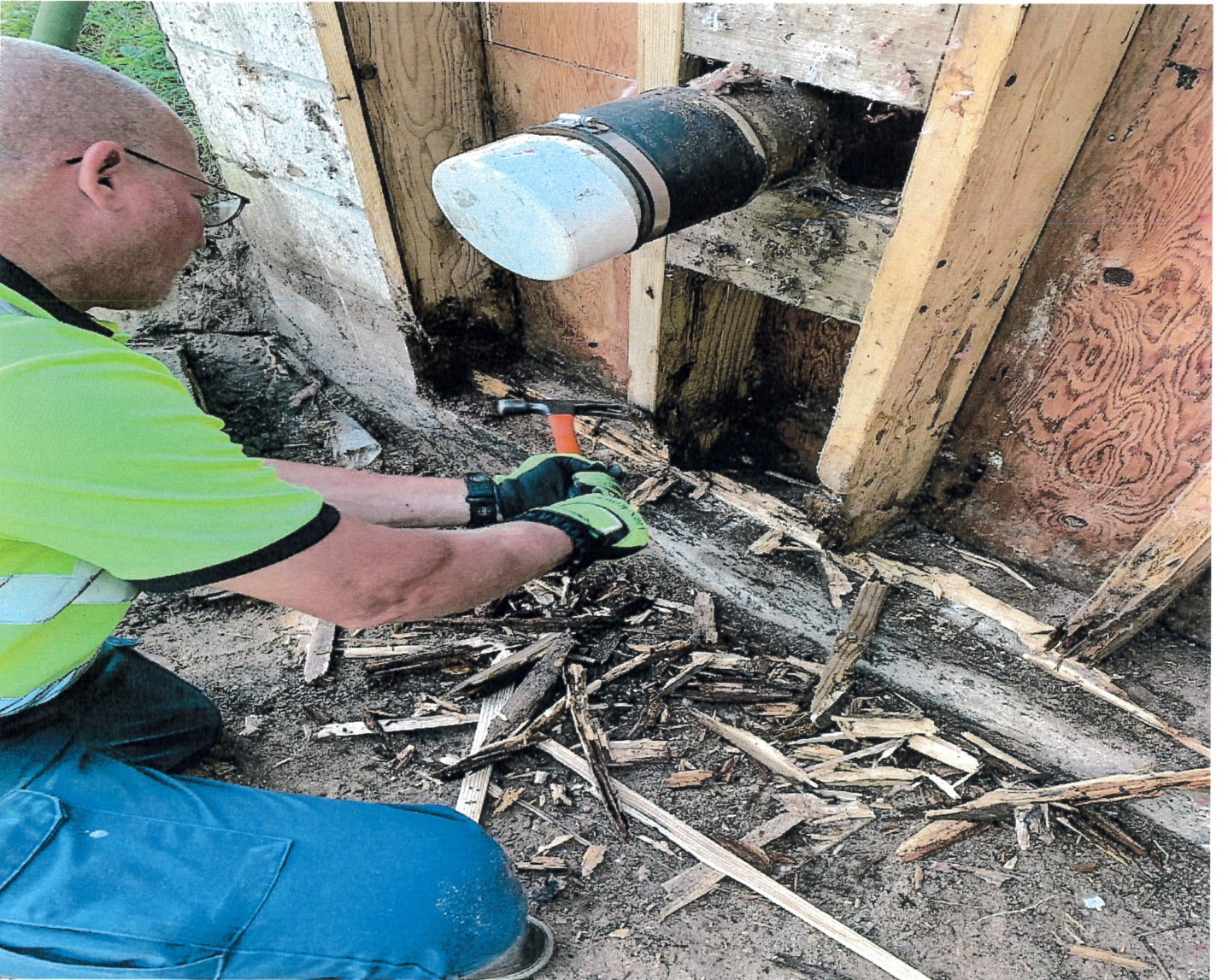
Wall is a total loss, severe damage from runoff infiltrating interior wall.
